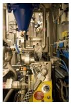
Due to the integration of a variable-frequency drive unit, the booster pump is now controlled as a function of demand so that the unit uses much less energy.
